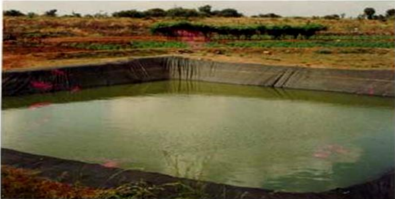
A farm pond lined with cotainment liner to control seepage
